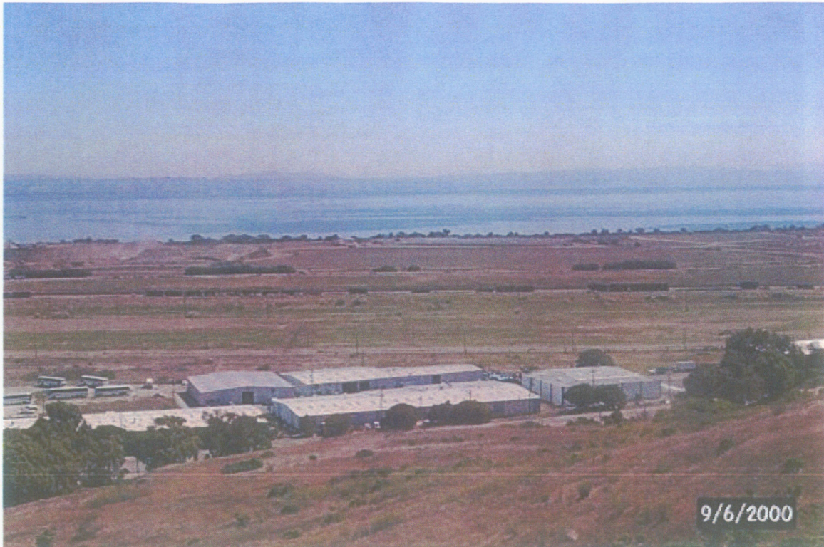
Central Baylands Subarea from Northwest Bayshore Subarea. Photo: Raphael Brien
